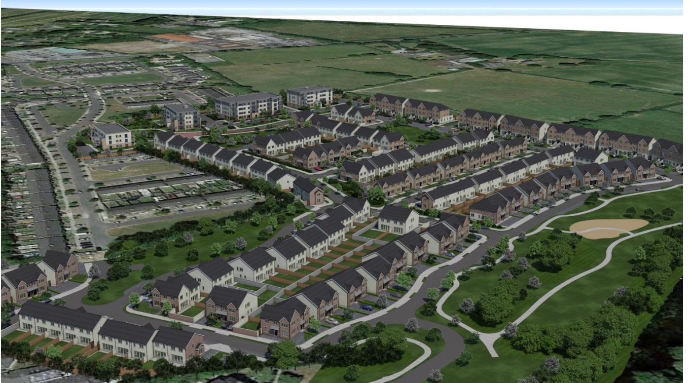
Fig 29: - Aerial View of the overall scheme from above the Liffey – Revised landscaping plan now incorporating the linear park along the river.
